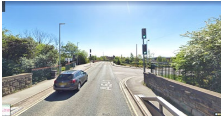
Mold Road Bridge : Constrained pavements. Railway access is screened. No framing to the either side of the street
