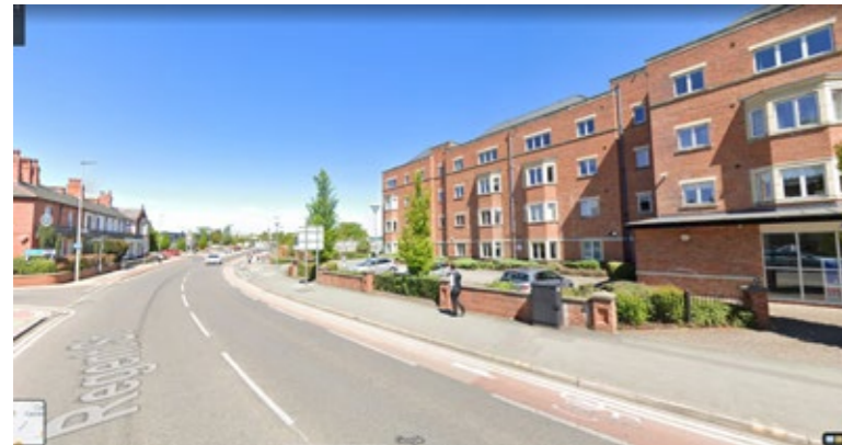
Regent street looking West 4 and 5 storey residential buildings define edge of town
